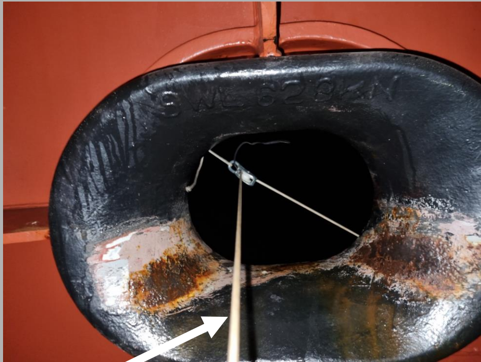
Rope from the winch
