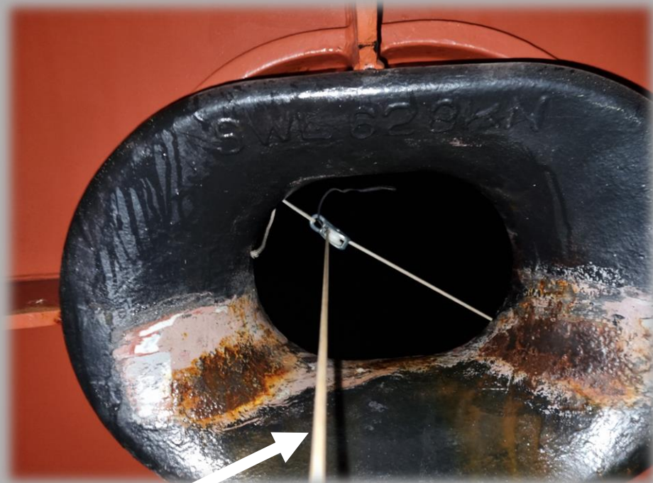
Rope from the winch
